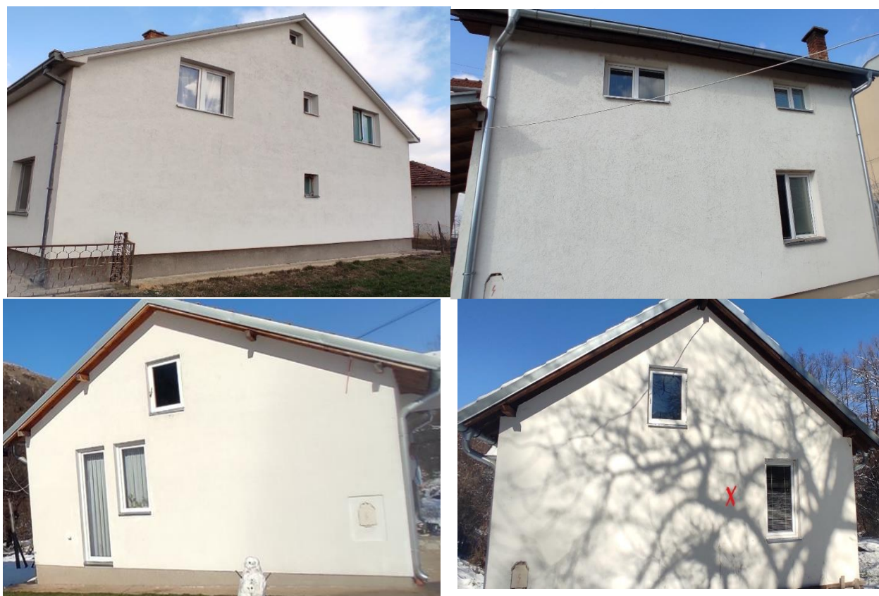
Picture 2: Photographs of differences in doors and windows
