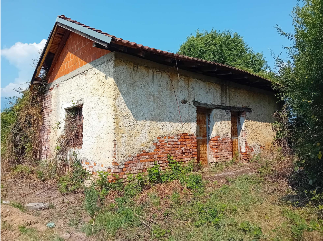
Photo 6: The facility where the pesticides are located.
