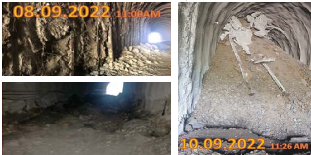
Picture 5. Tunnel 7 collapses - Picture from the supervisory body
