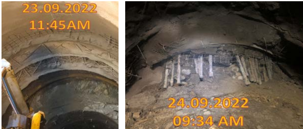
Picture 4. Tunnel 6 collapses – Picture from the supervisory body
